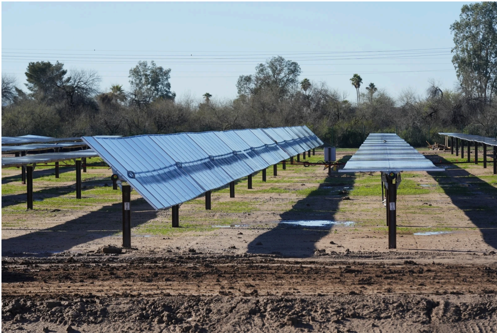
Rows of solar panels sit at Orsted's Eleven Mile Solar Center lithium-ion battery storage energy facility Thursday, Feb. 29, 2024, in Coolidge, Ariz. (AP Photo/Ross D. Franklin) Read More
